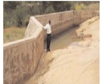
**The main requirement for making a rock catchment** is a rock outcrop with a large surface area.
